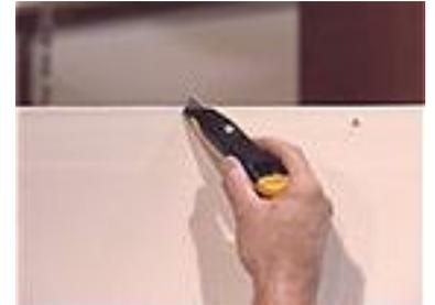
It's helpful to use a utility knife to score along the ceiling and all pencil marks before sawing out the damaged area.
