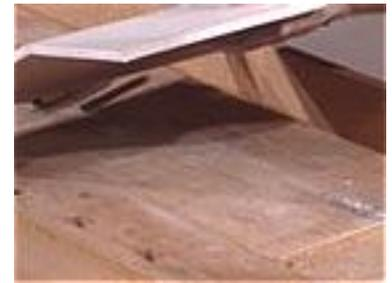
Score the drywall's paper with a knife, then simply snap the area to be cut out.
