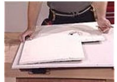
If the damaged area came out in one piece, use that section as a template when cutting a patch. Be sure to match the tapered area of the new piece with that of the old one.
